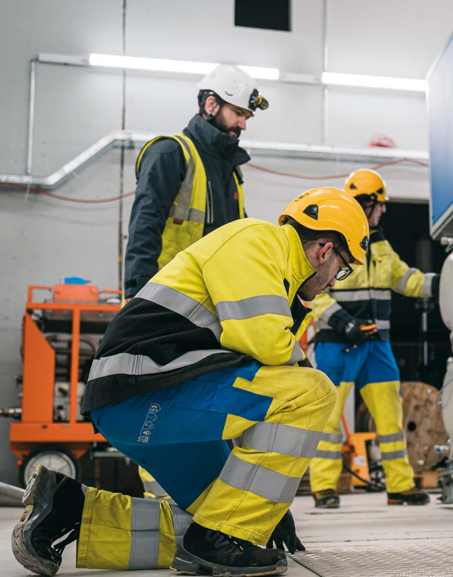
The switchgears allow to feed the energy produced by the Ritom and Stalvedro hydroelectric power plants into the 50 kV network, respectively to supply the railway network from the 50 kV network through the frequency converter.
