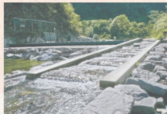
Details of the fish ladder
