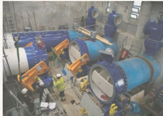
Overhaul of the Piottino plant
