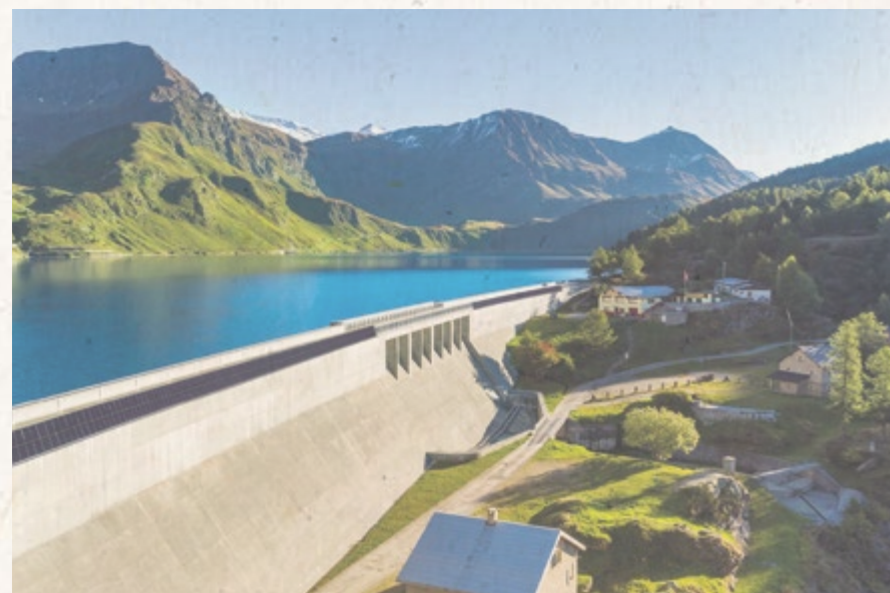
Project for the installation of a photovoltaic system on the Ritom dam
