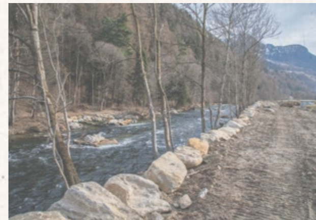
Renaturation of the embankment of the Airolo section
