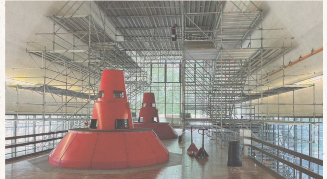
Restoration work on the vault of the Nuova Biaschina power station
